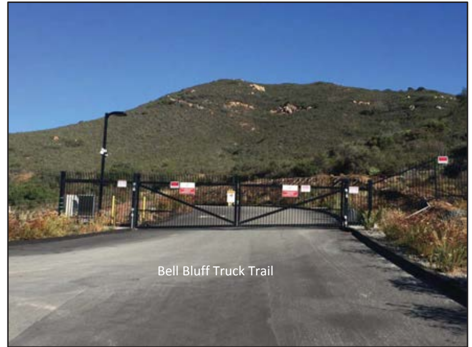
Photograph 2. View of electric gate on Bell Bluff Truck Trail road before Proposed Project site and SDG&E Suncrest substation property.
