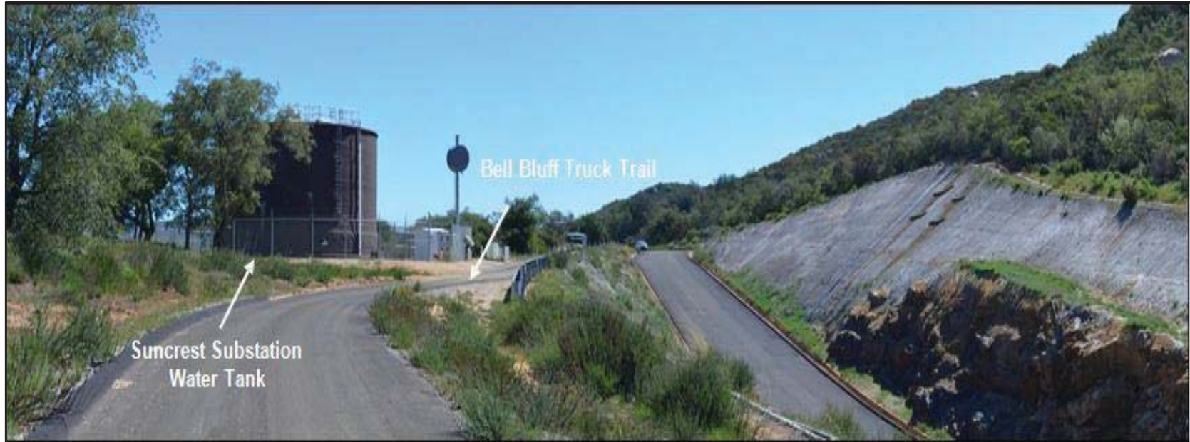
Photograph 11. View looking east at existing conditions with Suncrest substation water tank in foreground.
